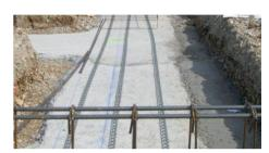
Strong and very resistant linear spacer, to be joined lengthwise and have several lengths. The new shape allows to combine high technical performances to a costs optimization.
