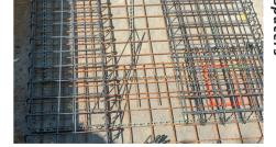
Spacer for horizontal use for heavy reinforcement and meshes; it withstands heavy incidental weights and loads with great stability.
