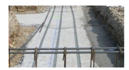
Strong and very resistant linear spacer, to be joined lengthwise and have several lengths. The new shape allows to combine high technical performances to a costs optimization.
