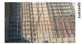
Spacer for horizontal use for heavy reinforcement and meshes; it withstands heavy incidental weights and loads with great stability.
